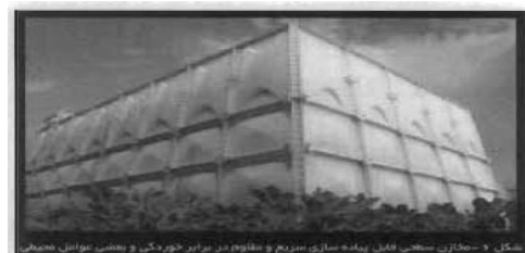
Figure6. Fast Implementable and Corrosion-Resistant Reservoirs
