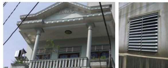
Figure1. The ventilation holes in tropical climates countries.
