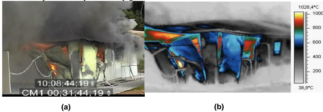
Fig6. Prototype after collapse: (a) camcorder view e (b) thermograph view.
