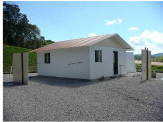
Fig1. General view of the prototype.
